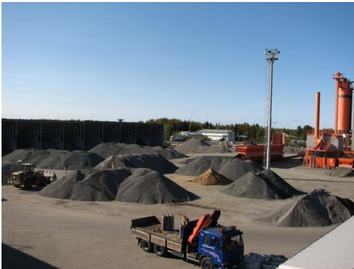
Figure 5.2. View of an asphalt plant, indicating possible sources of fugitive dust “This picture was intentionally chosen to be able to show the possible sources of fugitive dust. It is not intended to show the most perfect plant with regard to minimizing environmental and visual impact.”
