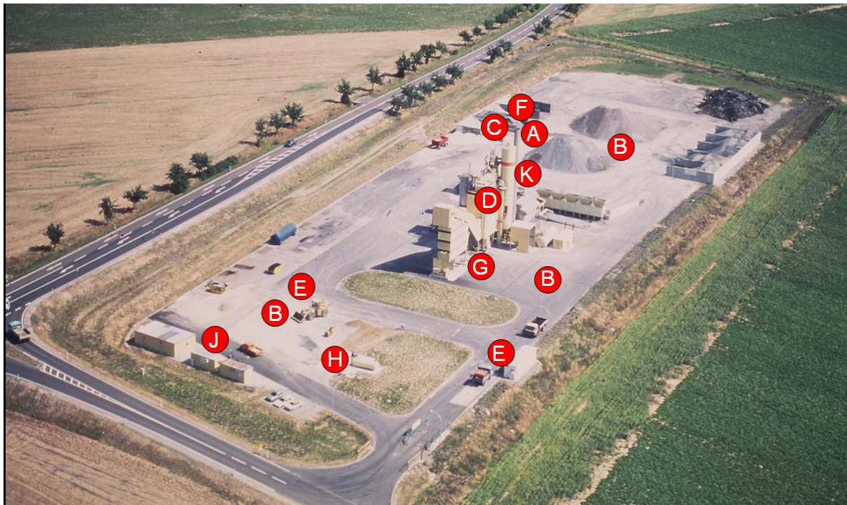
Figure 5.1. View of an asphalt plant, indicating possible sources of emissions. “This picture was intentionally chosen to be able to show all sources of emission. It is not intended to show the most perfect plant with regard to minimizing environmental and visual impact.”
